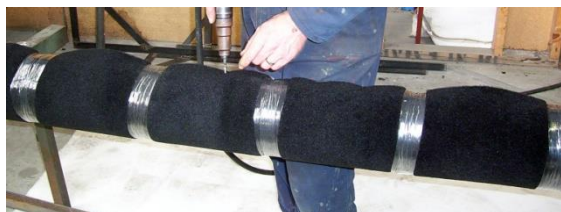
Fig 4 Starting to screw from centre
